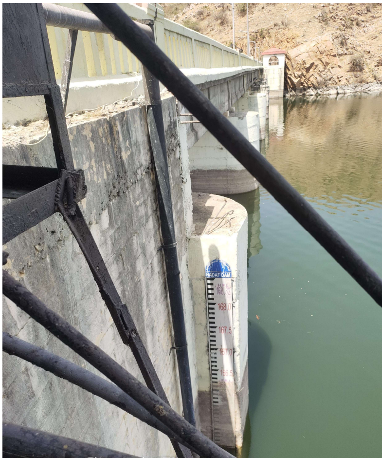
Photograph showing the Water Level Measurement Pillar at Hadaf Dam
